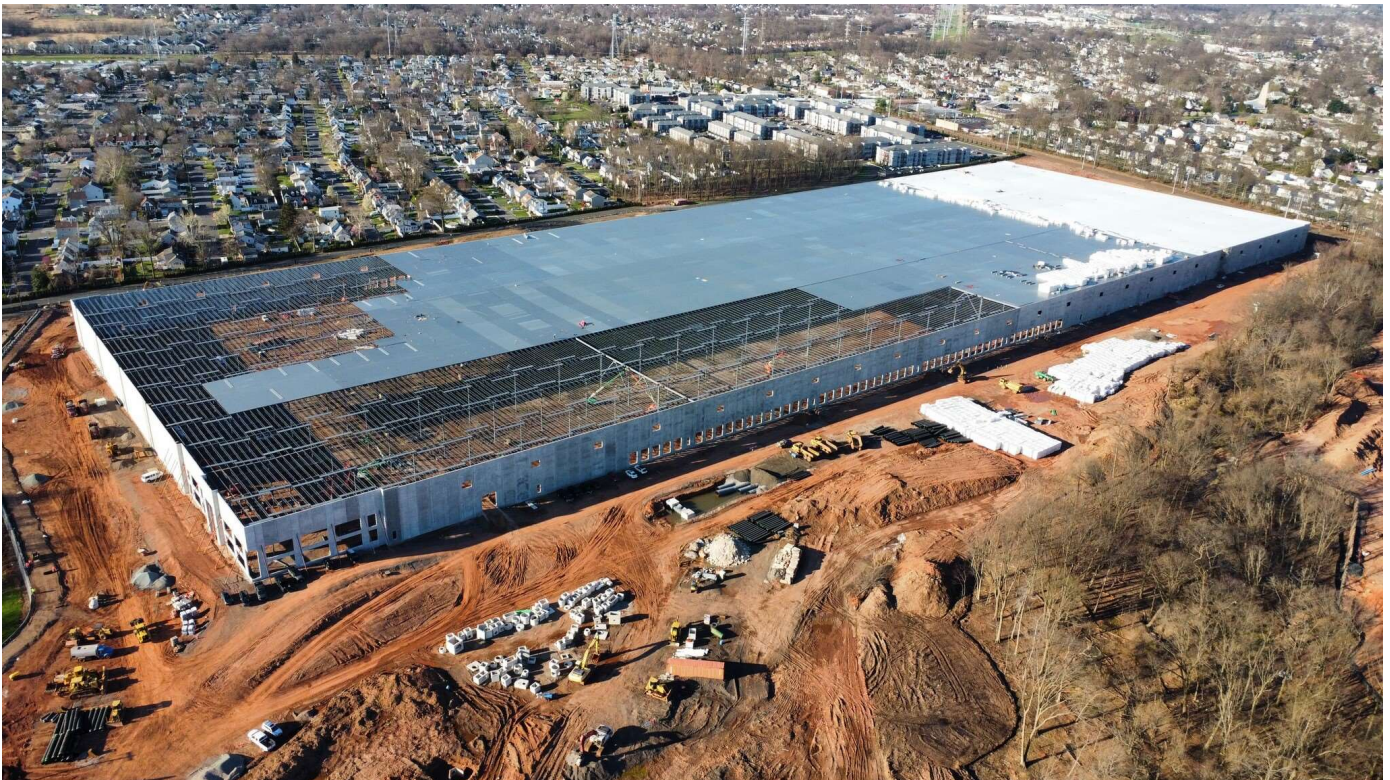
A logistics facility under construction in Rahway, New Jersey. (CoStar)
